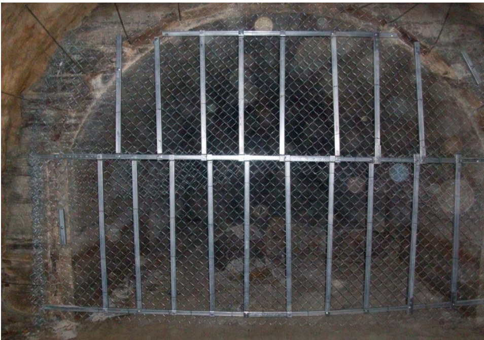
Barrier Wall Construction Completion.
