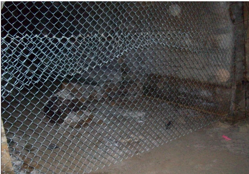
Chain Link Fencing Installation.
