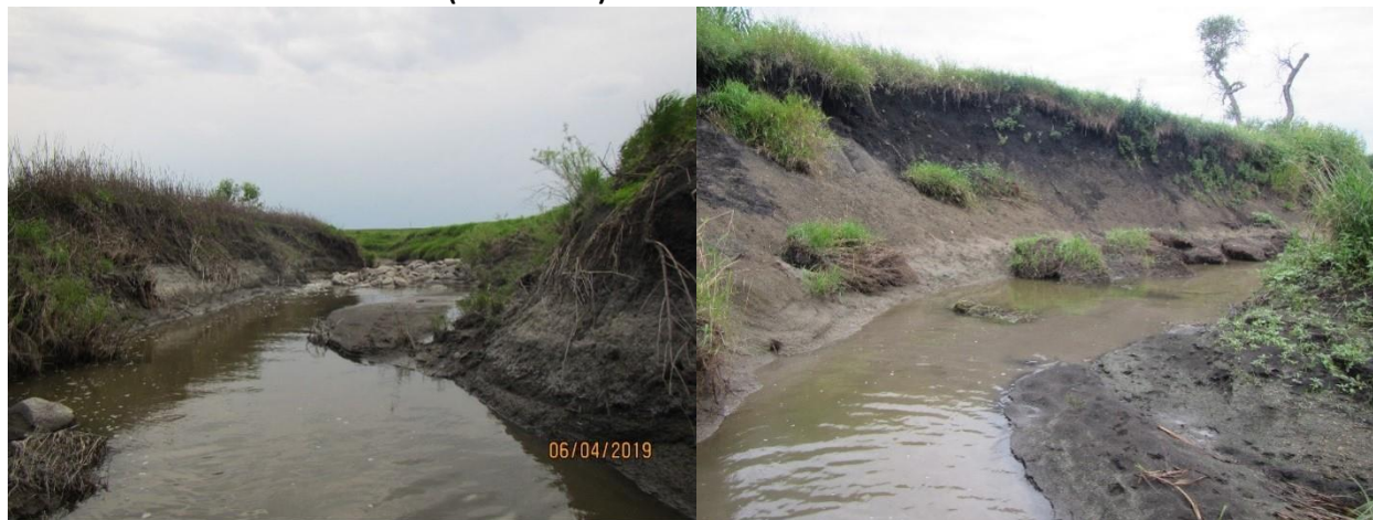
Figure 30. Bank erosion and instability documented in 2019 in Wolverton Creek (09020104-550) just downstream of 130 th Avenue South (MPCA 2023).
