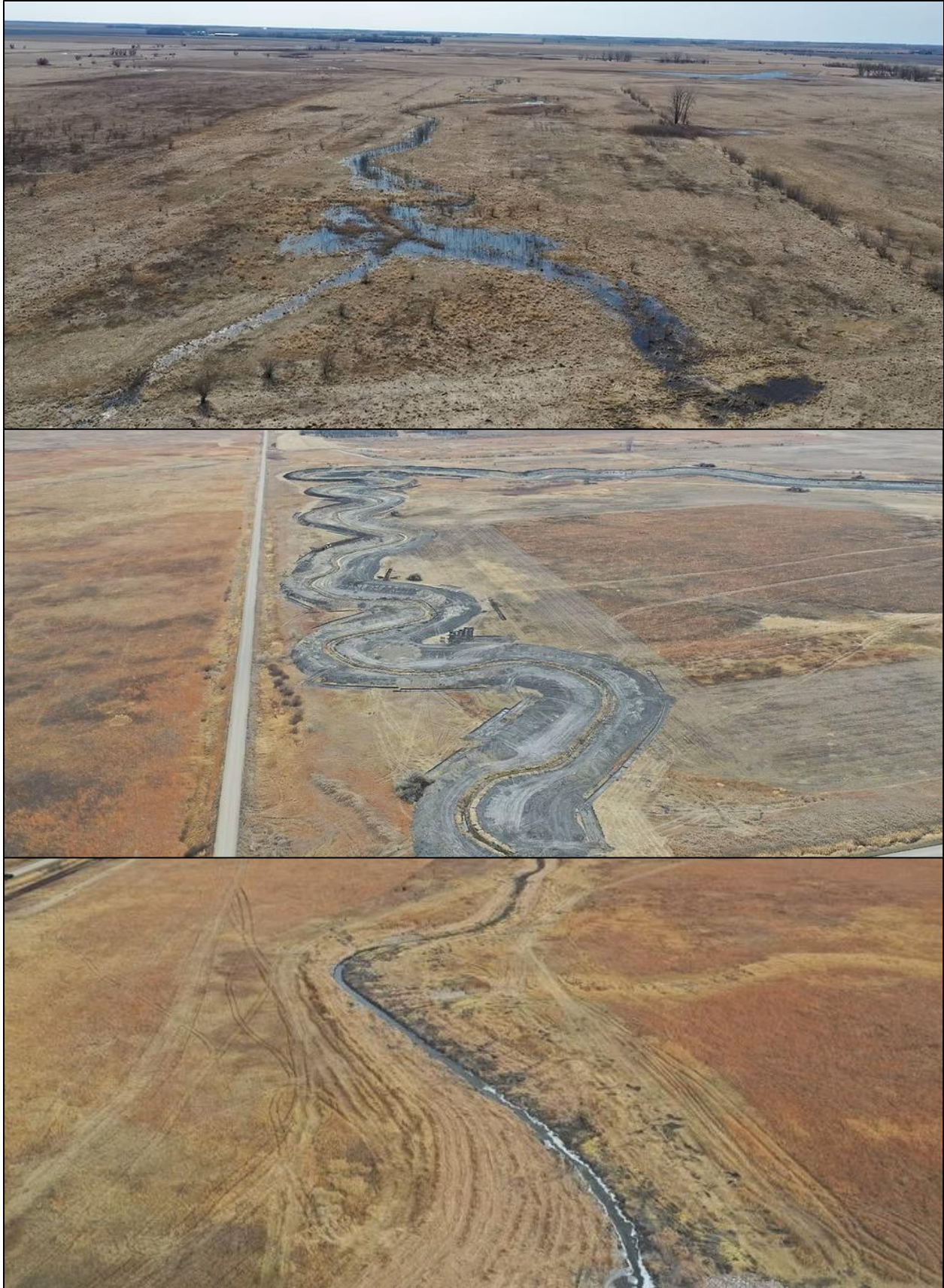
Figure 26. Pre- (top), during- (center), and post-project (bottom) photos of the Upper South Branch Buffalo River Restoration project phase 1 (BRRWD 2025a).
