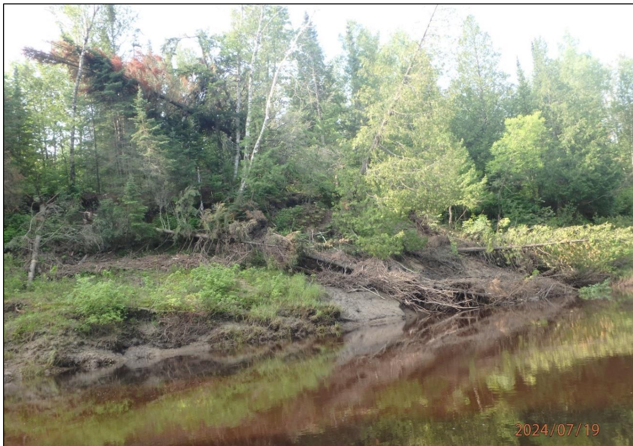
Figure 19. Mile 34.5 of the Little Fork Canoe Trail showing bank failure.
