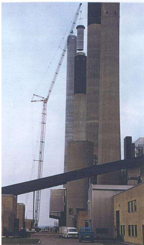
Figure 4: Installation of the chimney in 1995
