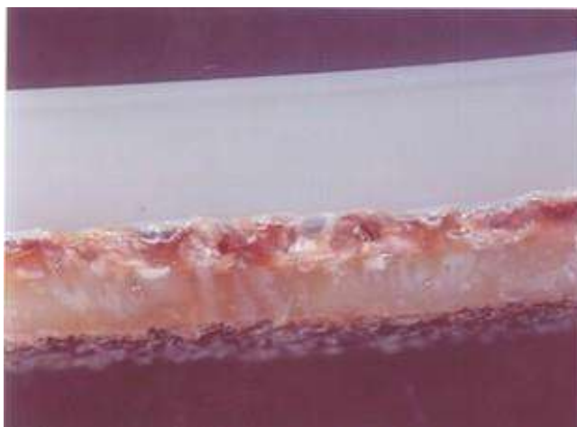
Figure 11: The cross section of the liner after 23 years of service
