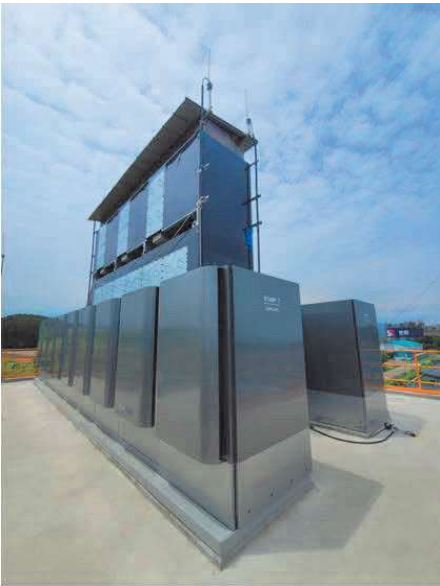
Figure 3: Bloom Energy’s heat capture installations
