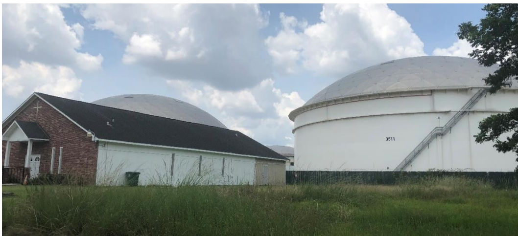
Source: Texas Environmental Justice Advocacy Services. View of aboveground storage tanks behind Groveland Missionary Baptist church in Pleasantville, 2019.
