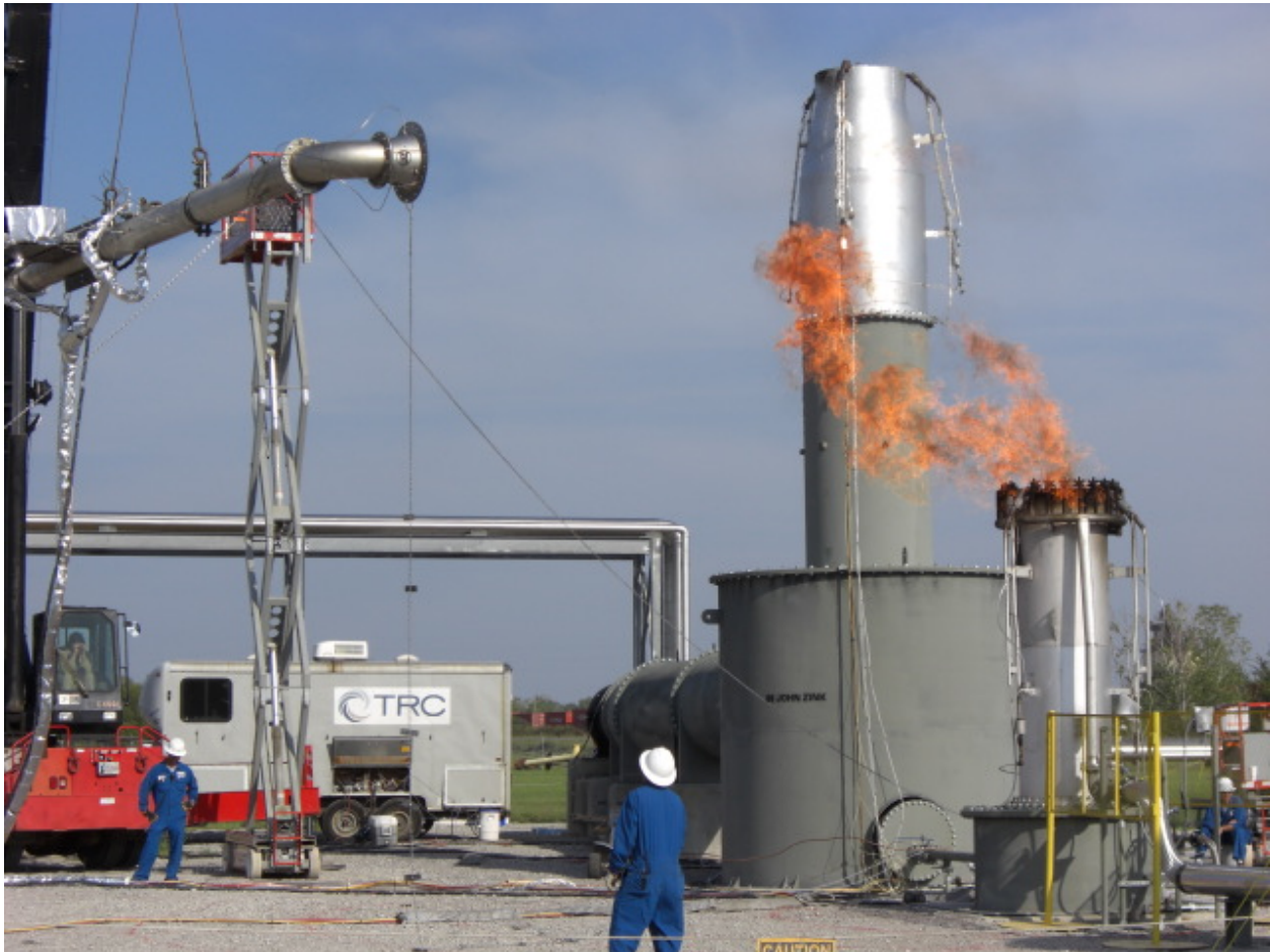
Figure 4-7. Flare Plume Sampling System. Plume sampling system making measurements of flare plume while held in position by crane and ground crew
