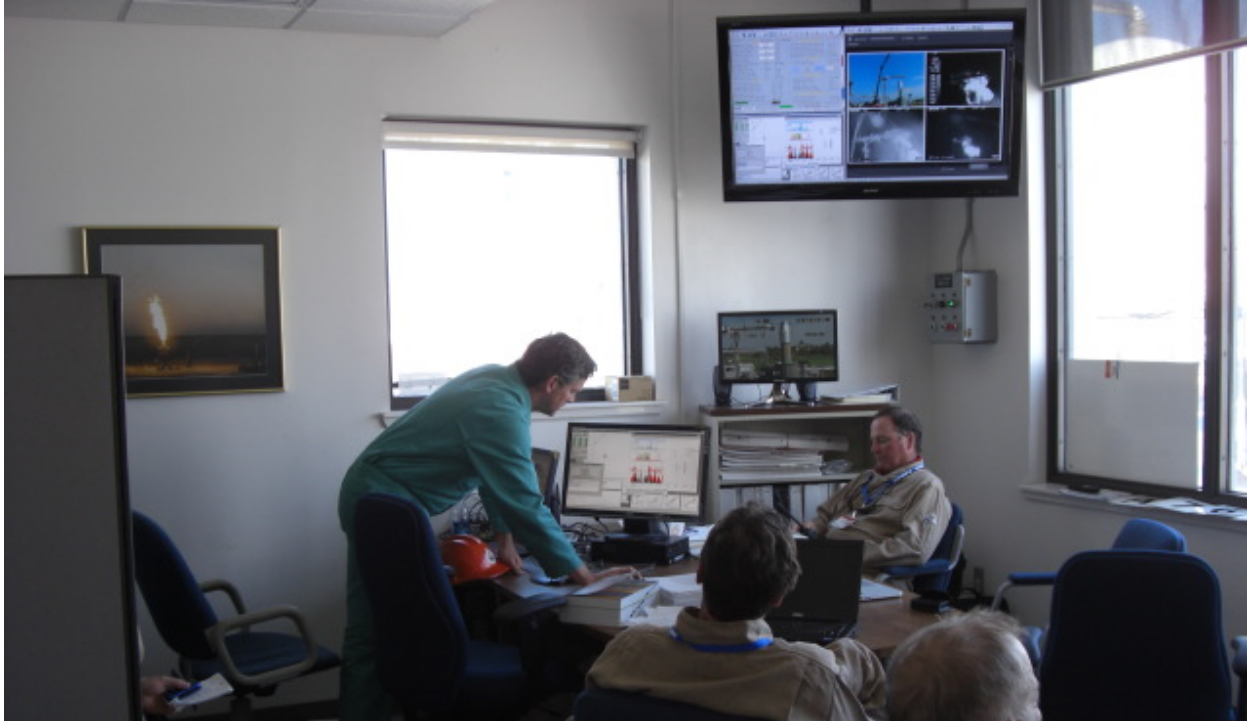
Figure 4-5. Control Room for the Flare Test System
