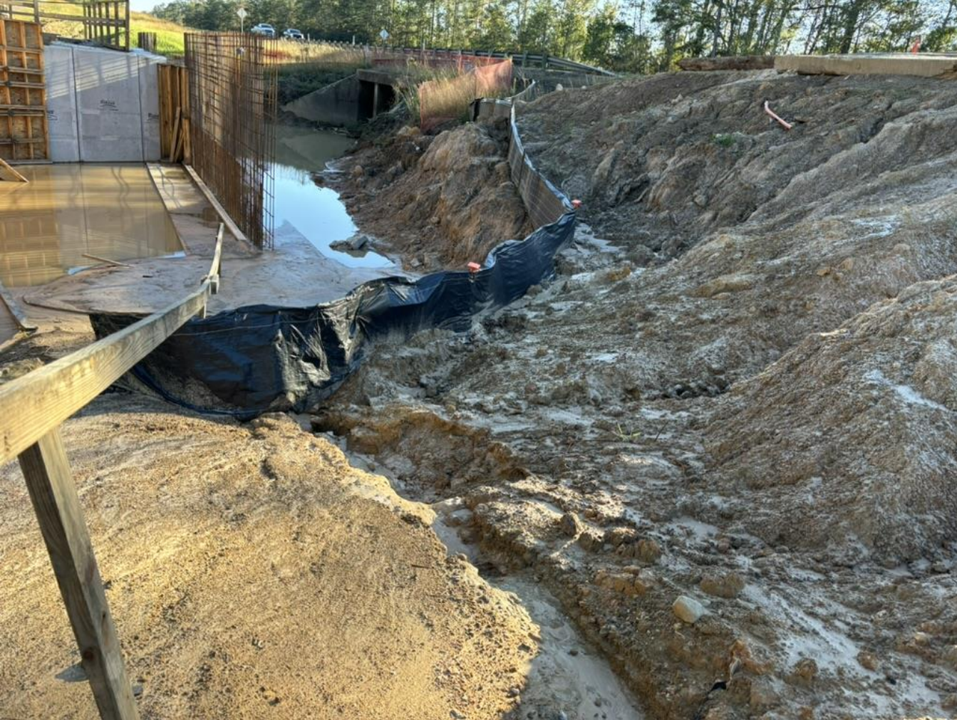
Erosion/sedimentation west side culvert 11-15-2024
