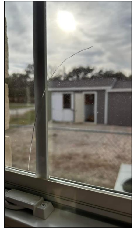
Figure 9. Broken Window from Quarry Blast. Source: CREAM
