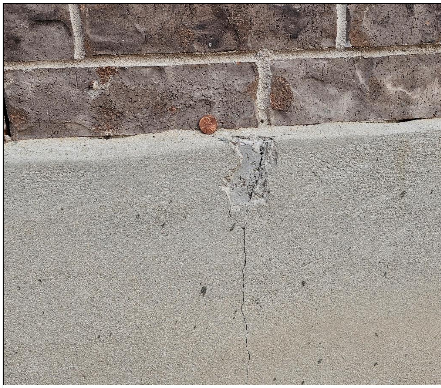
Figure 8. Crack in Foundation of House Near Quarry Blasts. Source: CREAM
