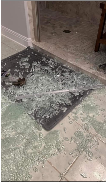
Figure 10. Broken Glass on Shower Door from a Quarry Blast. Source: CREAM
