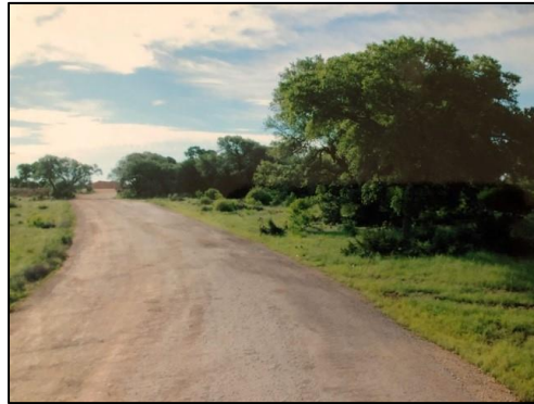
Figure 20. Vegetation and Trees Used to Control Dust on Haul Roads. Source: Jill Shackelford
