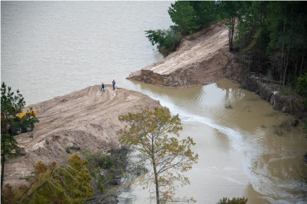
Broken dike at the Triple PG sand mine in Porter. Industrial wastewater is flowing out of the mine into White Oak Creek which joins Caney Creek and the San Jacinto East Fork before flowing into Lake Houston.
