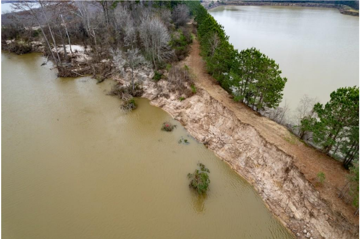
Dike of abandoned Williams Brothers Mine (upper right) eroded by the San Jacinto West Fork (lower left).
