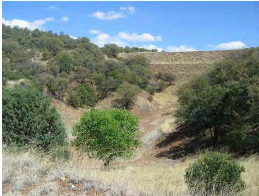
View of tailing pile no.4, looking upstream; this pile is the second and lowermost of the two piles proposed for installing the evaporation ponds. Note steep sided nature of this pile, showing the need for additional reinforcement (buttressing) to support additional weight of ponds
