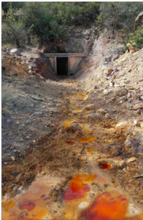
Figure 2. The adit at Lead Queen Mine, before remediation.
