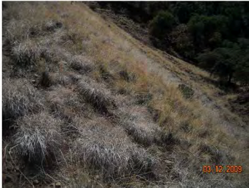
Close-up of side slope of tailings pile no. 4 showing the steep-sided nature of the tailings impoundments' slopes
